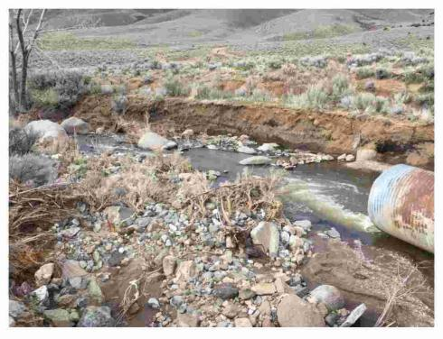
Downstream damage to creek from Washed out Culvert
